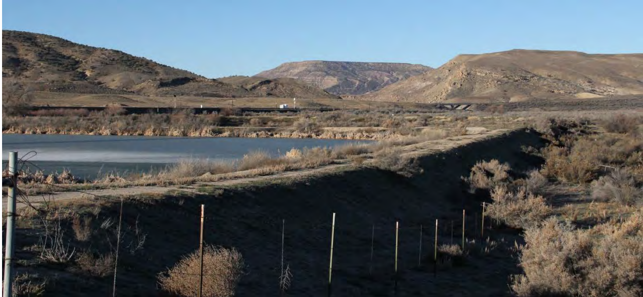
Photo C-13. UP Connection Point, MP 0.0 of Alternative 2 at Mack, Colorado. UP main track is in background. Looking railroad-west toward the entrance to Ruby Canyon and the Colorado River.
