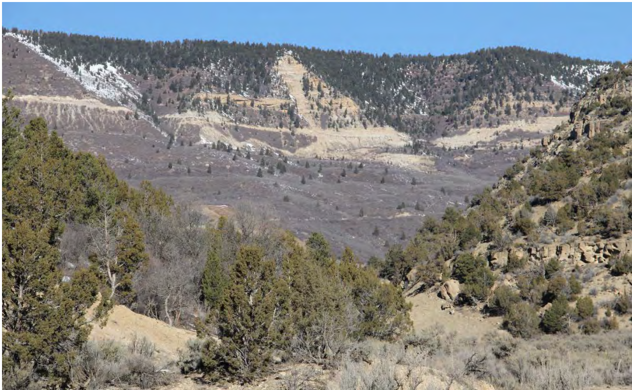
Photo C-15. Baxter Pass above Atchee, Colorado, MP 28.5±, Looking Geographic West. The alignment of the old Uintah Railway is visible crossing the face of the ridge, ascending from right to left using a 7.5% grade. Note the large landslide area crossing the Uintah Railway grade that has broken out to the ridge line near the middle of the photograph. The hummocky area below the old Uintah Railway grade appears to be a sizeable landslide.
