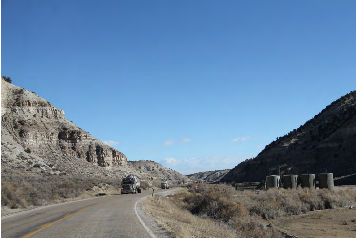
Photo C-5. Looking North (Railroad-East) in Indian Creek Canyon near MP 36 of Alternative 2.
