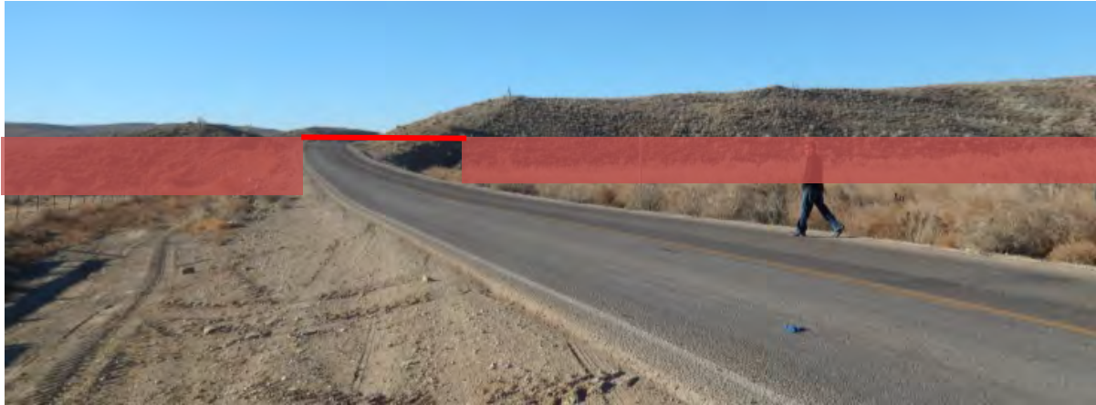
Photo C-17. Common Segment MP 1.0 Crossing Sowers Road. View is looking south on Sowers Canyon Road. Red shaded area shows approximate height of railroad embankment.
